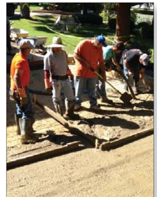
Alex and his crew lay a new driveway.
